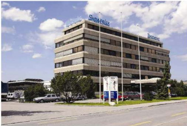
Head Office, Switzerland
